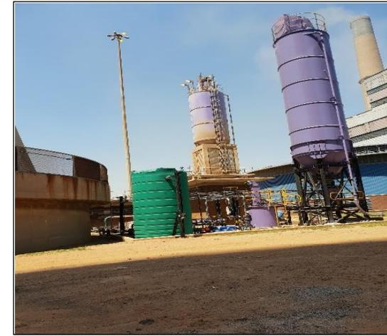
Silo's and a mixing tank on the existing Lime Treatment Plant at the Kriel Power Station
